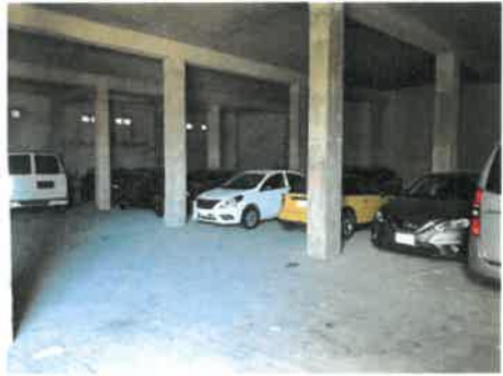
Typical Warehouse Interior (2020)
